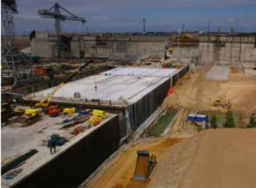
Figure 5: Tunnel construction beneath S1 navigation opening
